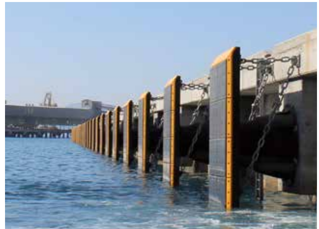
Container Terminal | Aqaba | Jordan
